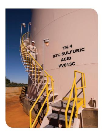
Proper venting of storage tanks is essential to dissipate any hydrogen evolved. Potential sources of ignition (such as sparks and flames) should be excluded from the vicinity of the storage tank to minimize the fire or explosion hazard from hydrogen generation.
